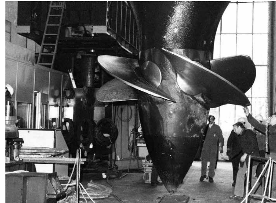
August 1918 - Work in progress on the Kaplan rotor in the Hône 1 power plant
