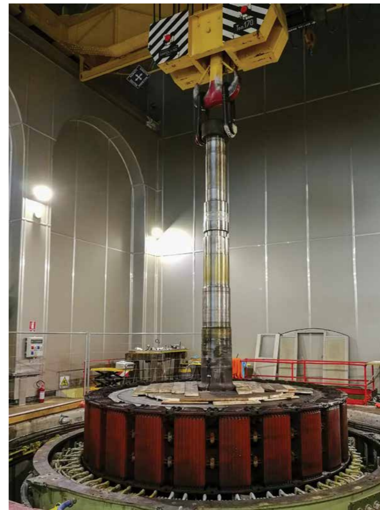
Rotor extraction of the Hône 1 power plant
