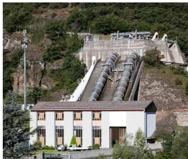
Montjovet power plant
